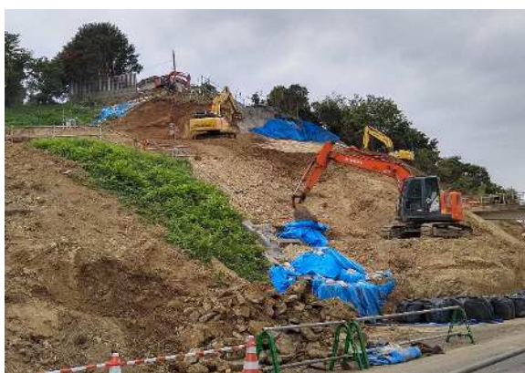
③崩落土排土
