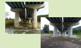
橋梁の耐震補強
